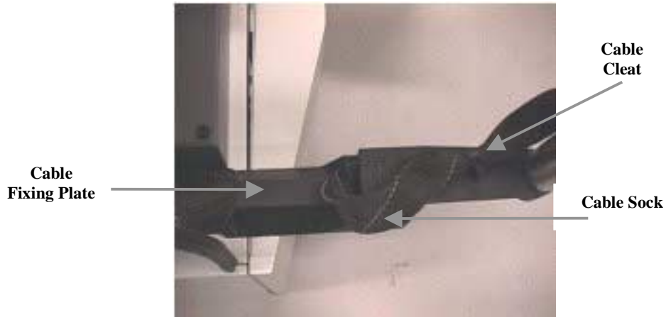
Figure 2.18 Cable Fixing Plate and Cable Sock
